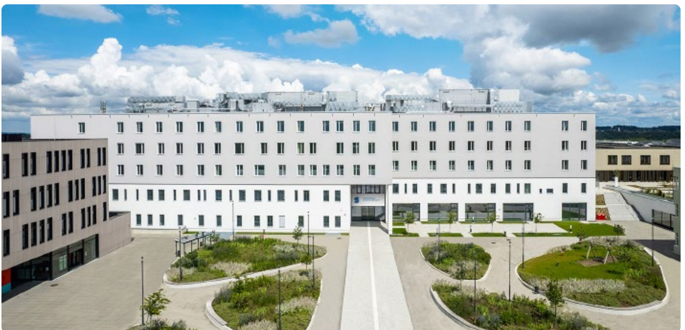
On the way to the Smart Hospital: The new building of Sana Klinikum Biberach
